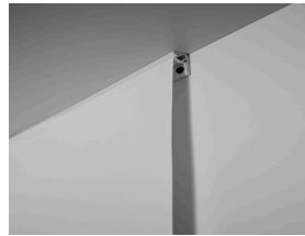
Clipso wall installation with PCC profile.
